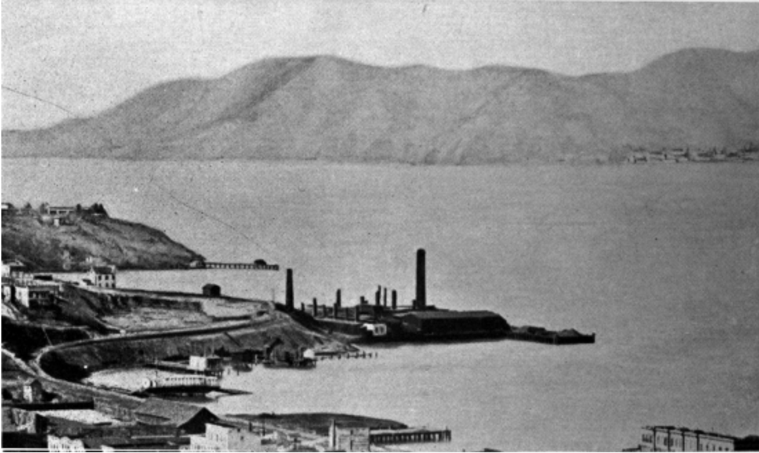
"The Golden Chimney."
