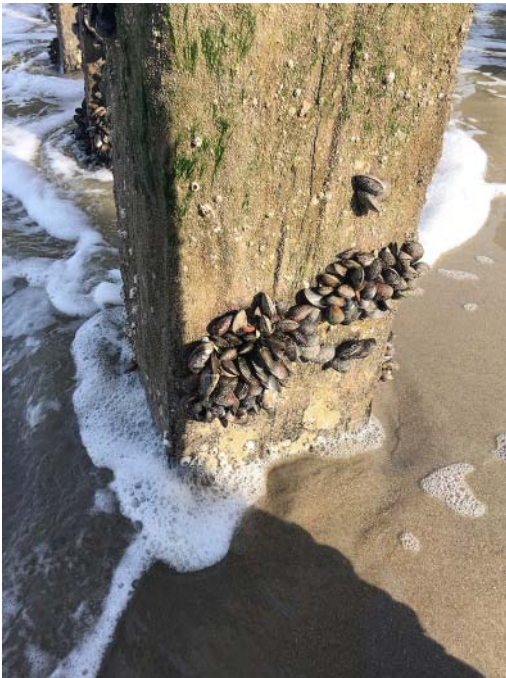
Figure 1.5 Mussels adhesive bonded to a wooden pile in the North Sea near Domburg, the Netherlands. Source: Dr. Jürgen Klingen, Aboso-Consulting.
