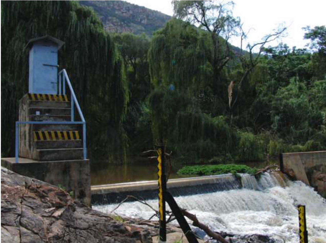
View of surface flow and water quality monitoring station A2H049 at the lower end of the Bloubank Spruit at Zwartkop showing hut housing automated stage gauging instrumentation at left, and vertical stage gauge plates in middle and right foreground for visual observation; the blockage by vegetation and debris of the left flank of the weir (right of picture) is not ideal; the northern slope of the 1626 m amsl Zwartkop peak forms the backdrop to this view ( Photo P. Hobbs, date 05/02/2010 )
