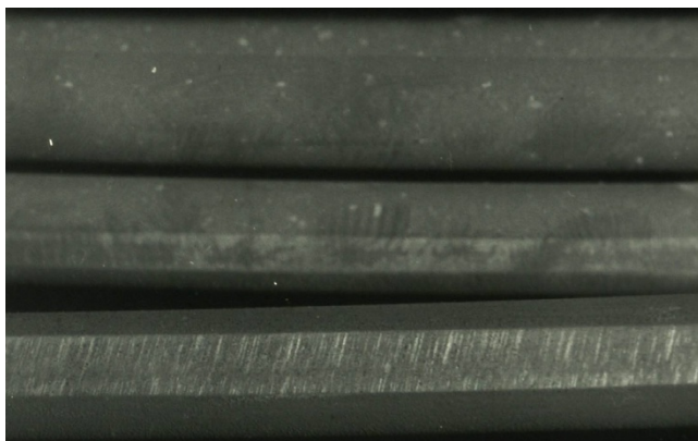
Fig. 1-1 Tube-to-Tube Fretting Wear in the U-Bend Region of an Early Nuclear Steam Generator (Pettigrew, 1976).
