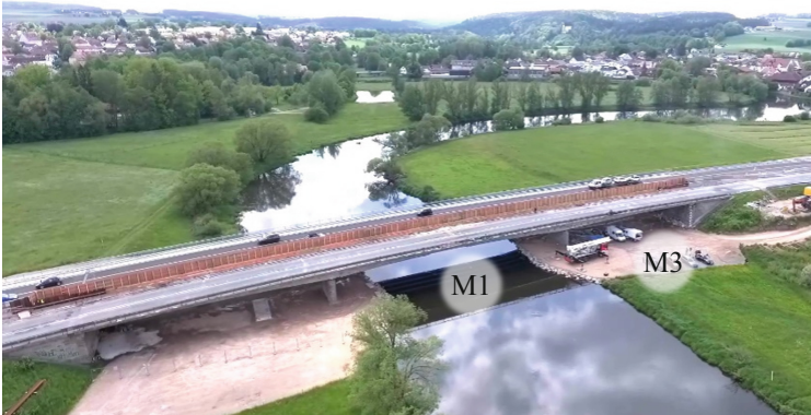
Fig. 1. Overview screen of the trial bridge in Roding
