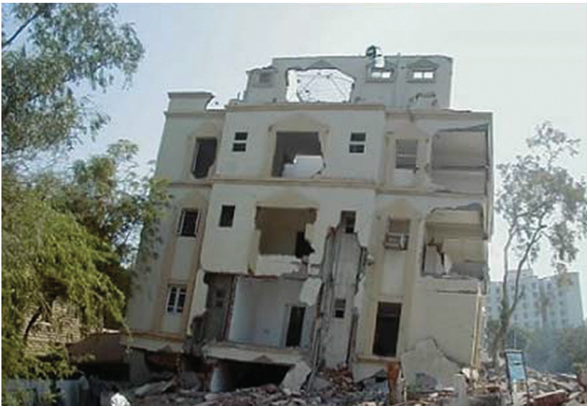
Figure 2.3 Reinforced concrete building in the Kutch district and typical damage patterns. Notice ground floor failure.
