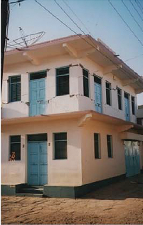
Figure 2.2 Brick masonry building with reinforced concrete floors damaged in the Bhuj earthquake.
