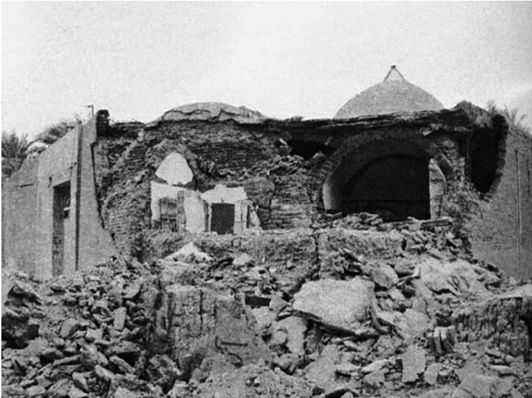
Figure 2.6 Failure of adobe dwelling in the Bam earthquake. Source: World Housing Encyclopedia. Reproduced with permission of EERI.
