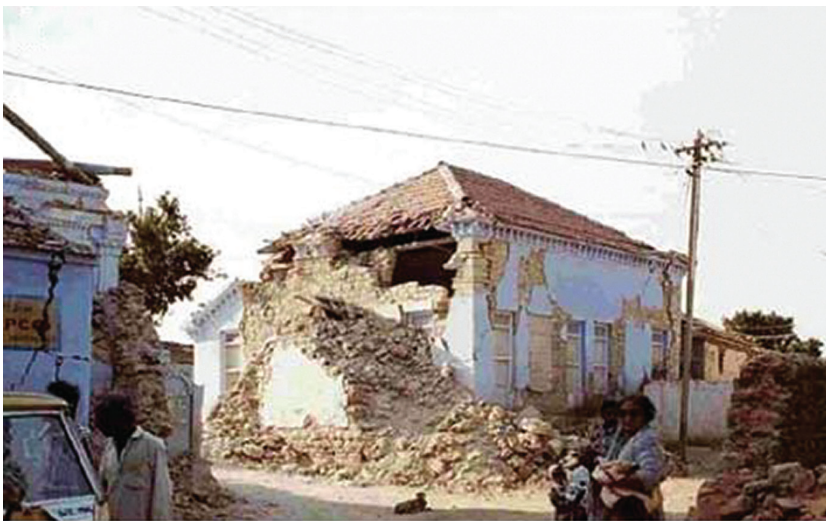
Figure 2.1 Stone masonry building in the Kutch district damaged in the Bhuj earthquake.
