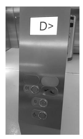
Fig. 1 Destination call control for an elevator (own image)
