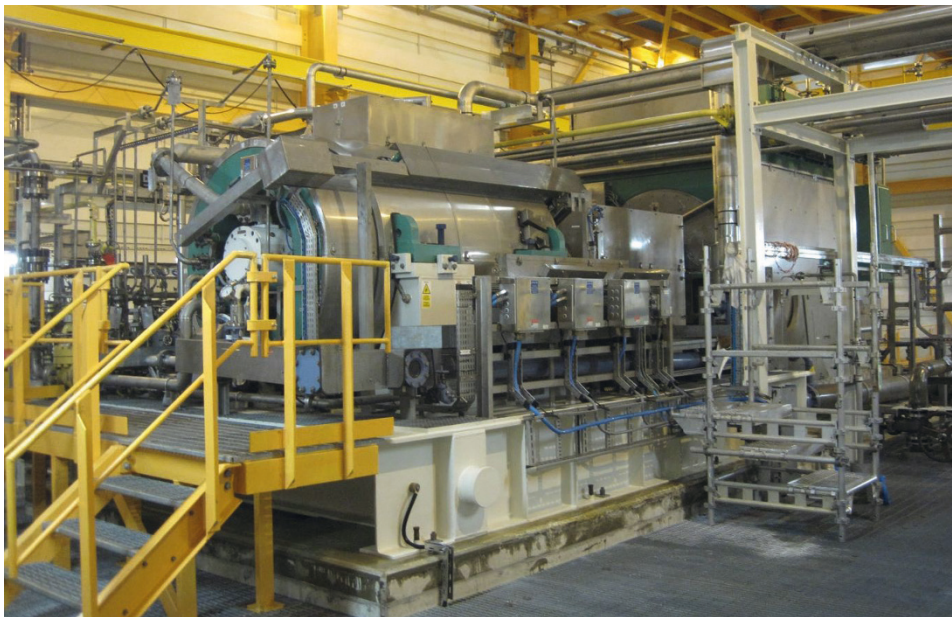
Optimizing torque control for a multi-megawatt compressor.
