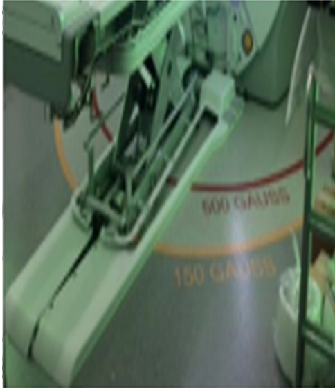
Figure I.3 The 5 Gauss line. A scan room floor.
