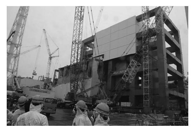
*The steel structure for the use of the spent fuel removal from the cooling pool is seen at the Unit 4 of the Fukushima Daiichi nuclear plant at Okuma in Fukushima prefecture, Japan.*
