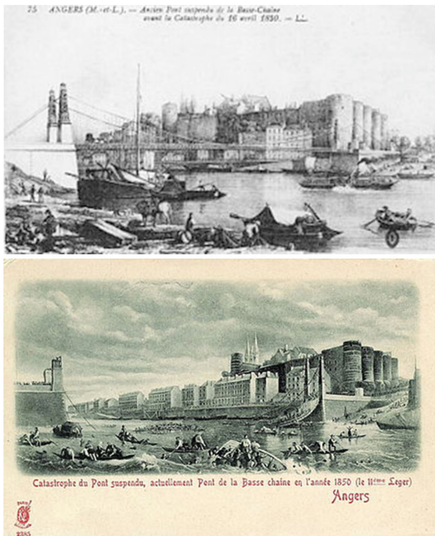
Fig. 7 The bridge over the river La Loire in France which collapse in 1850: before (above) and after (below)
