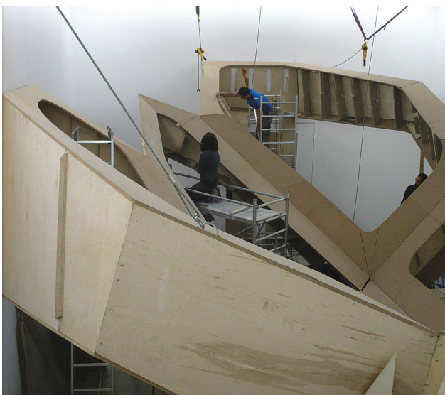
Views from construction in Portikus. Photos: Luis Etchegorry
