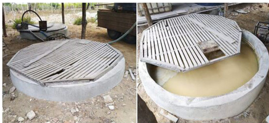
Fig. 1 Cassava wastewater storage tank
