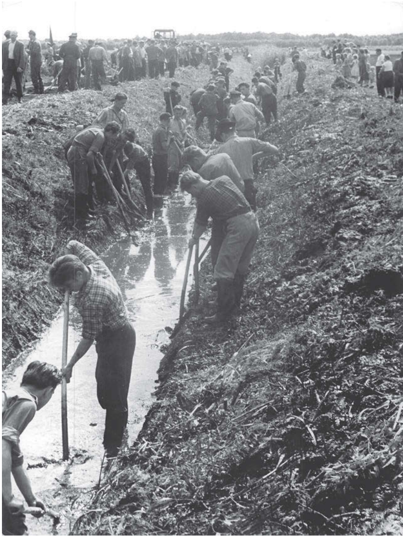
Figure 2.2: Adolescents digging a drainage ditch in the Friedländer Große Wiese, Germany (Zentralbild Schwankler, 11.8.1958).
