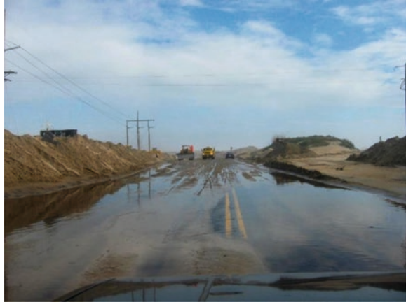
Fig. 1.11 Highway 12 on Pea Island, North Carolina, looking north showing an eroded dune on the right and bulldozed sand on the left during a nor'easter. (Image by S.J. Culver)
