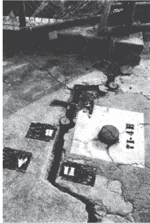
Figure 1.1.8 Two-inch separation between Pacoima Dam Arch (left) and the thrust block (right) on the left abutment (Scott et al. 1995).
