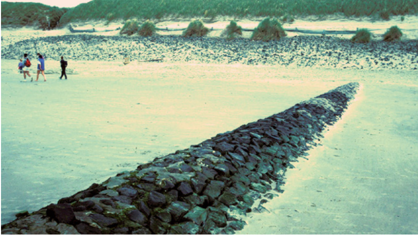
Figure 1.9 Large groin to protect the beach from erosion on the North Sea coast of the Netherlands. There is a small dike landward of the dry beach.
