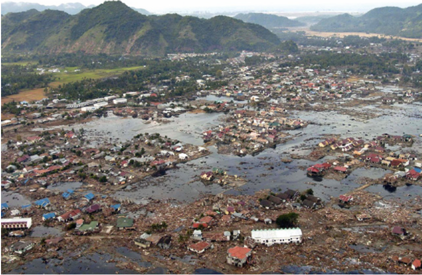
Figure 1.13 Photograph of the devastation near the coast of Japan where the 2011 tsunami came ashore.
