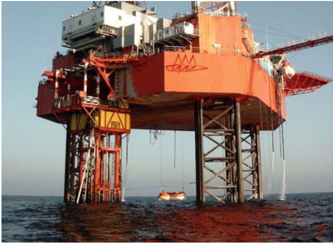
Fig. 1.21 An oil rig
