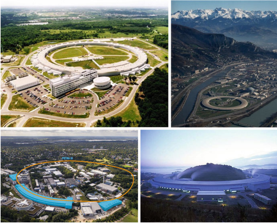
Fig. 1.6 The four largest storage ring dedicated synchrotron radiation sources in the world. Top left: the Advanced Photon Source (APS) at Argonne National Lab near Chicago. Top right: European Synchrotron Radiation Facility (ESRF) in Grenoble, France. Lower left: PETRA-III in Hamburg, Germany. Lower right: SPring-8 near Osaka in Japan
