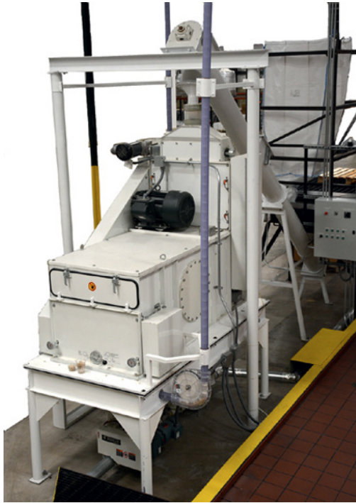
Figure 1.3 Mill at Susquehanna Brewing Company.
