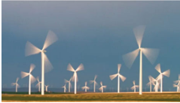
Picture 1.2 Few realize wind turbines are inherently unsustainable and nowhere close to being renewable.
