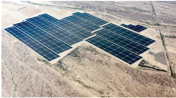
Picture 1.1 This big solar project in Arizona is just one of the large clean power plants enabled by the Energy Department's Loan Program Office. Credit: Courtesy of NRG.
