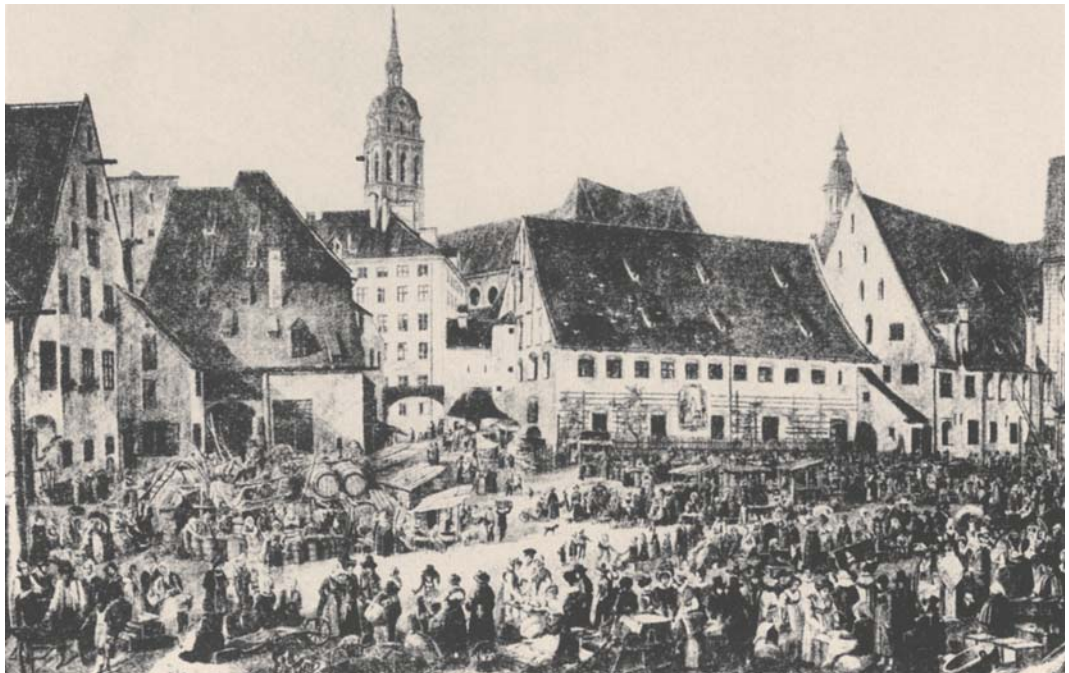
■ Fig. 1.3. View of the Hospital of the Holy Ghost in Munich (from H. Kerschensteiner, 1913). On the right-hand side of the picture: end of the nave of the Holy Ghost Church; the view over today's fruit and vegetable market shows the tower of the old town hall and the old St. Peter's church. In front were the units for men and for women. Approx. at the position of the observer were the »idiot pits«.
