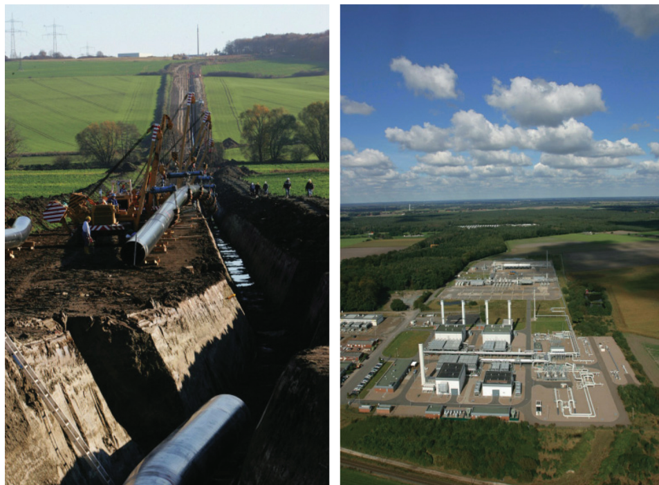
Figure 1.3 Left: Building a natural gas pipeline in Eastern Germany. Right: Storage facility for 4.2 billion m 3 of natural gas in Rehden, 60 km south of Bremen. Source: Photos: WINGAS GmbH.
