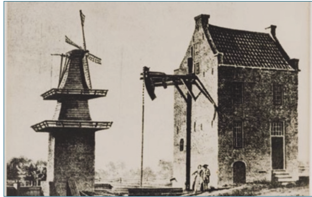
↑One of the very first steam engines ('fire machines') in The Netherlands was built in Heemstede (near Haarlem) in 1781. It had to replace the windmill on the Groenendaal estate which had been unable to pump enough irrigation water. (courtesy of Noord-Hollands Archief)
