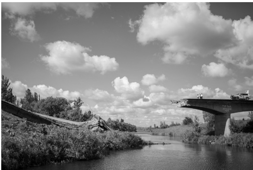
Figure 2: Ukraine, destroyed bridge in Sloviansk (© Photothek)
