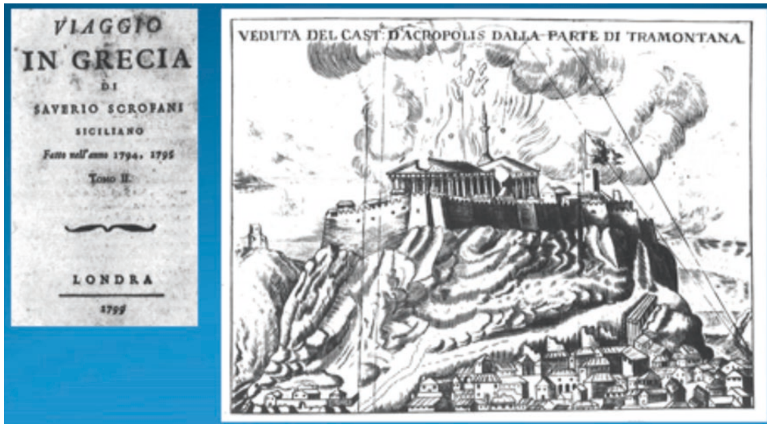
Fig. 2.8 In 1687 a shot of mortar fell the Parthenon
