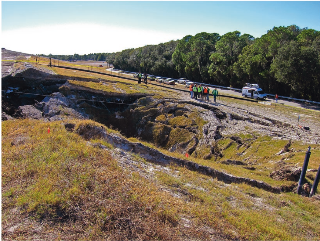
Fig. 1.4 Collapse failure of a landfill over a sinkhole at the Southeast Hillsborough Landfill near Wimauma, Hillsborough County in 2010. Site, which has been remediated, was located at 27.776°N, 82.188°W. People provide scale
