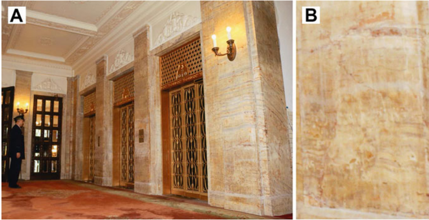
Fig. 1.1 “Onyx Marble” in the Japanese Diet Building. (a) Elevator hall. (b) Closeup image of a column showing laminated texture. (Image was provided by Kitaniippon Newspaper Co. Ltd.)
