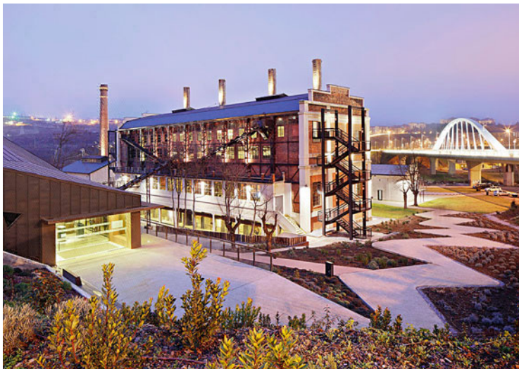
Fig. 2 Ponferrada’s “La Fábrica de Luz. Energy Museum”, an award-winning rehabilitation of the one-century old thermal power plant. Published with the kind permission of the author, José Hevia, through the good offices of Míriam Fernández Cuevas
