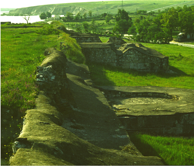
Fig. 2: Capidava in Scythia Minor, looking north along the eastern curtain wall.
