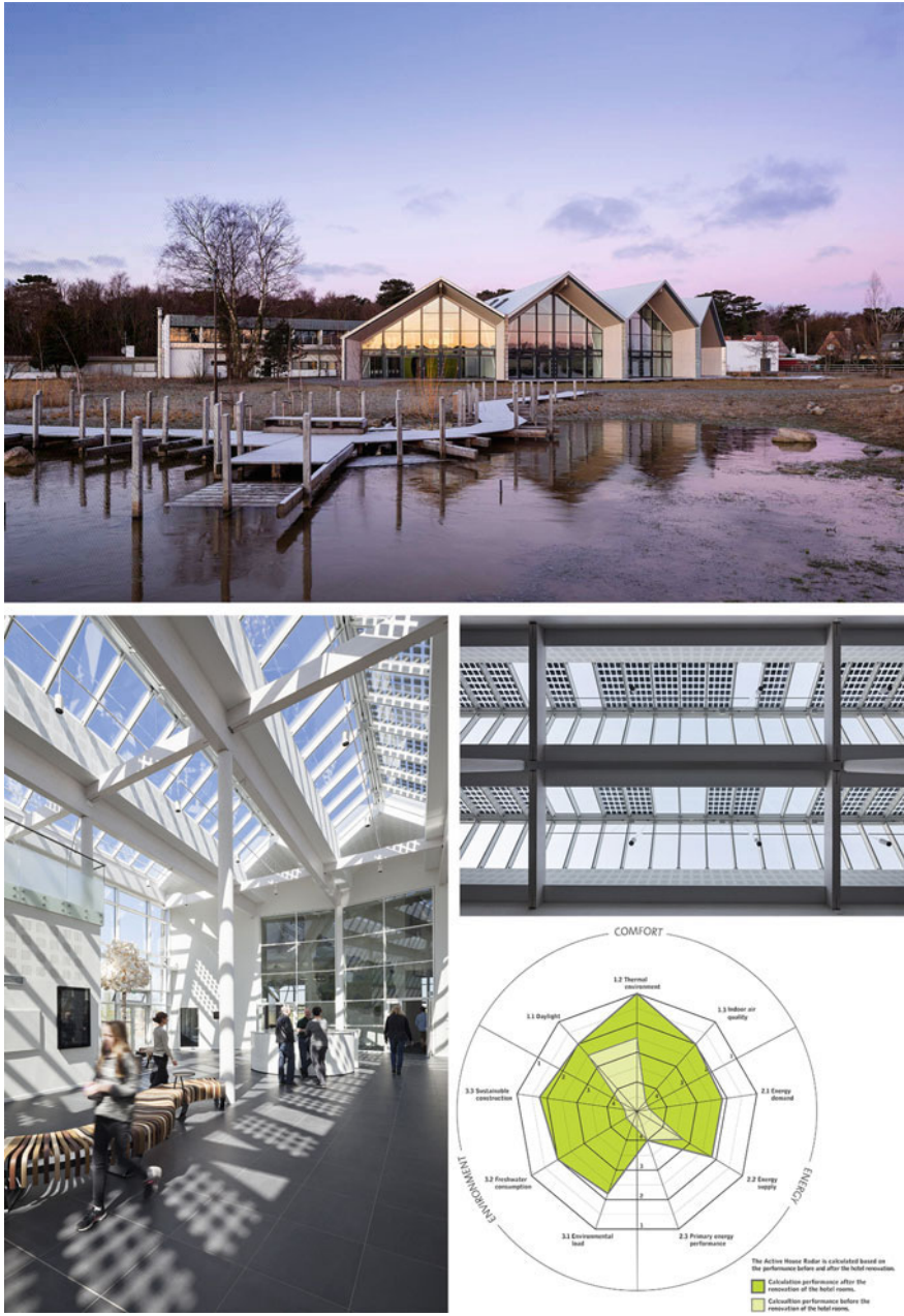
Fig. 1.1 The Green Solution House is an example of Active House labelled projects; its design integrates Active House principles and applies Active House specifications, as shown by the Active House Radar of the project (Ph. Adam Mørk, AH Radar © Adam Mørk)
