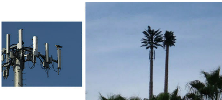
Fig. 1.1 Examples of cellular base station antennas are shown. LHS is a closeup view of antennas, and RHS is another example where antennas are blended as part of tree in an attempt to be less visible to the environment. Antennas are most visible part of the whole cellular infrastructure equipment
