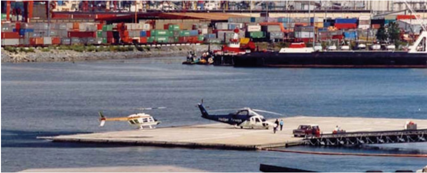
Fig. 12 Floating helipad supported by geofoam blocks in Vancouver, Canada ( www.mansonvilleplastics.com )
