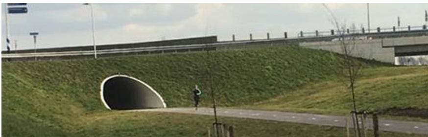
Fig. 28 Finished structure (InfraDelft)
