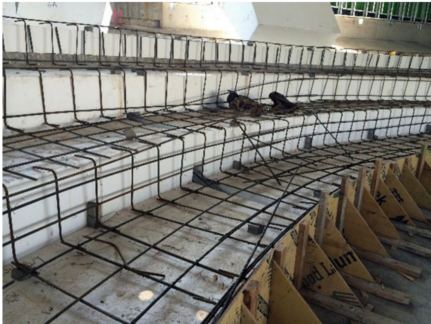
Fig. 15 Stacked Geofoam blocks for seating arrangements ( http://blog.achfoam.com/?p=2455 )
