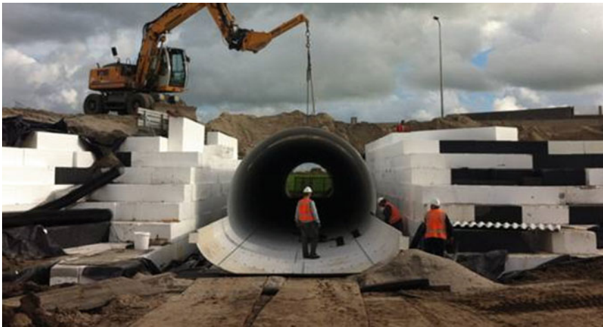
Fig. 27 Construction of corrugated steel tunnel in EPS fill (InfraDelft)
