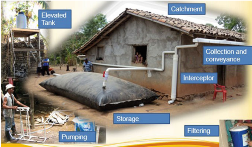
Fig. 6 Roof catchment connected to a geomembrane bag in Honduras. Source Kadet (2017)
