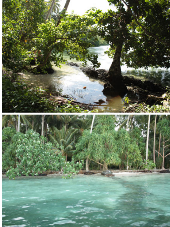
“Gabion baskets”, wire-enforced structures filled with rocks on the Island of Han, Tulun Atoll. (Photos taken in 2010 by Luetz)
