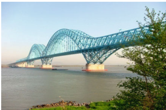
Fig. 1.7 Nanjing Dashengguan Yangzi River Bridge
