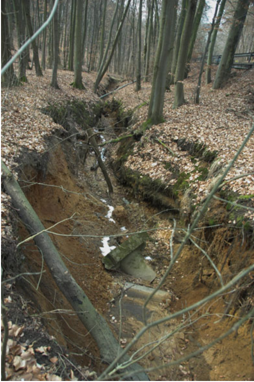
Fig. 1.9 Up to 5 m deep incised active gully in a sandy valley fill near Kopstal (west of Luxembourg city) as a consequence of concentrated discharge of surface water, the front part of the concrete tube itself is eroded (photo BK)
