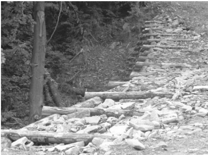
Fig. 2.7 Reconstruction of forest roads with local materials (Photo: Edward Pierzgalski)
