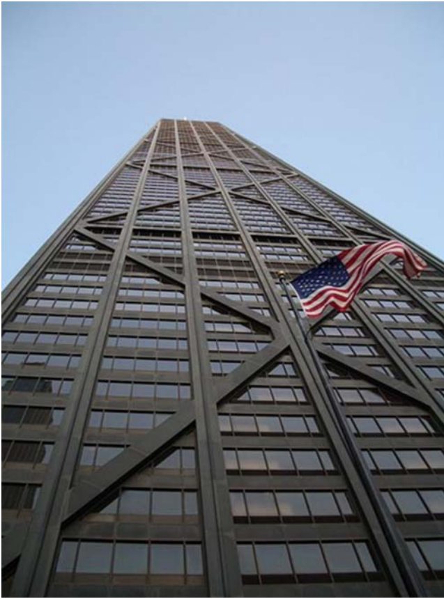
Figure 1.2 Braces emphasized esthetically in the John Hancock Tower of Chicago. Source: From Wikipedia; photo courtesy of "Akadavid", 2008.
